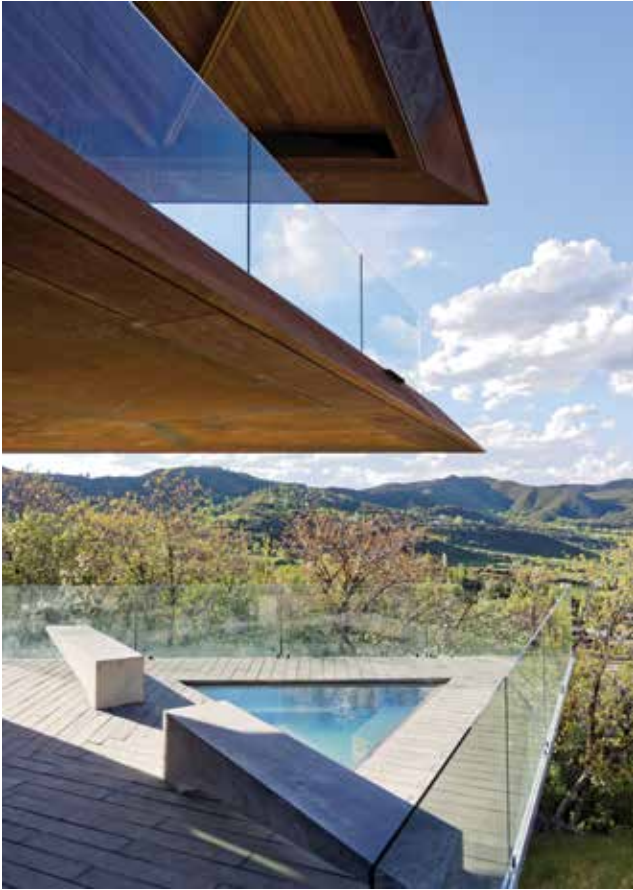
The triangular spa mirrors the cantilevering above. The deck is made from ipe wood. Photo: Stephen Miller
